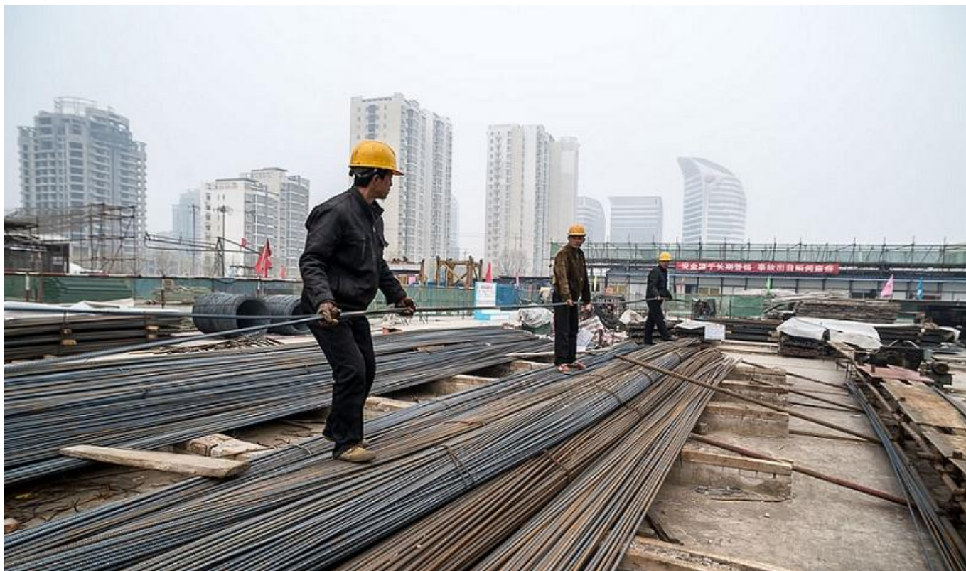
Construction workers in Beijing, March 2013. Photo by Joe Tymczyszyn / Creative Commons
